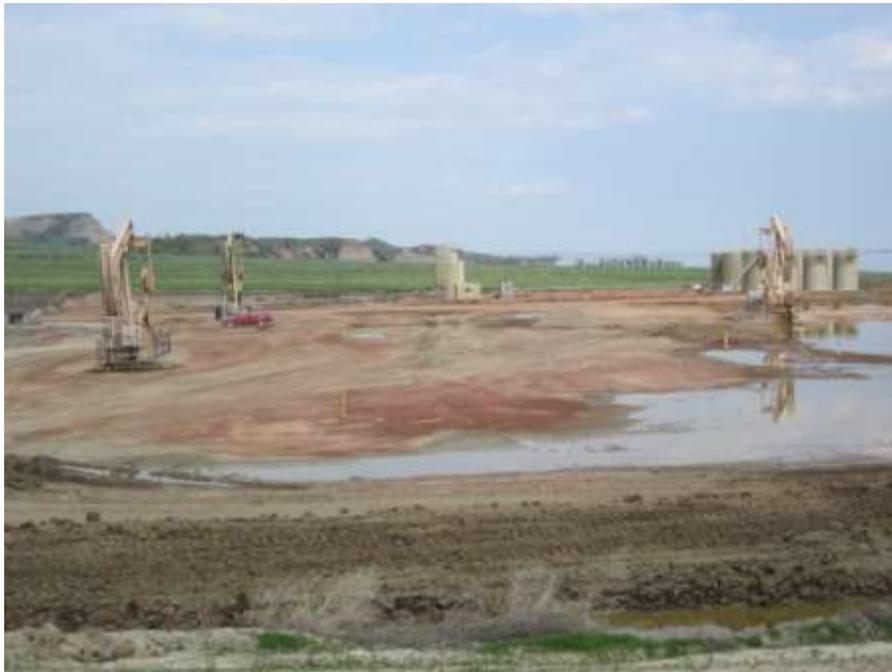
Photo 3. Hofflund Wildlife Management Area along Lake Sakakawea/Missouri River. Mega-pad well site being diked to prevent rising reservoir levels from flooding the well pad on June 4, 2011. Reserve pit is buried in the left foreground.
